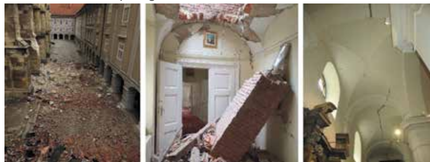
Figure 32. Damage to the cathedral's parish house and the St Mary's Church (source: Ministry of Culture of the Republic of Croatia and [39])
