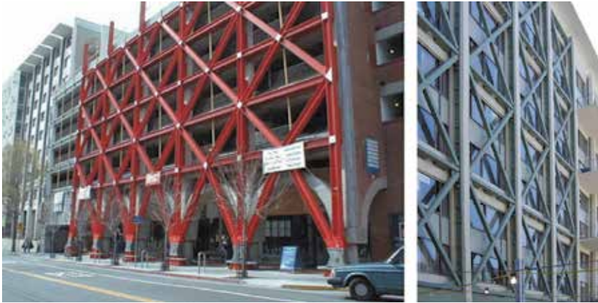
Figure 8. Buildings retrofitted with external steel braces
