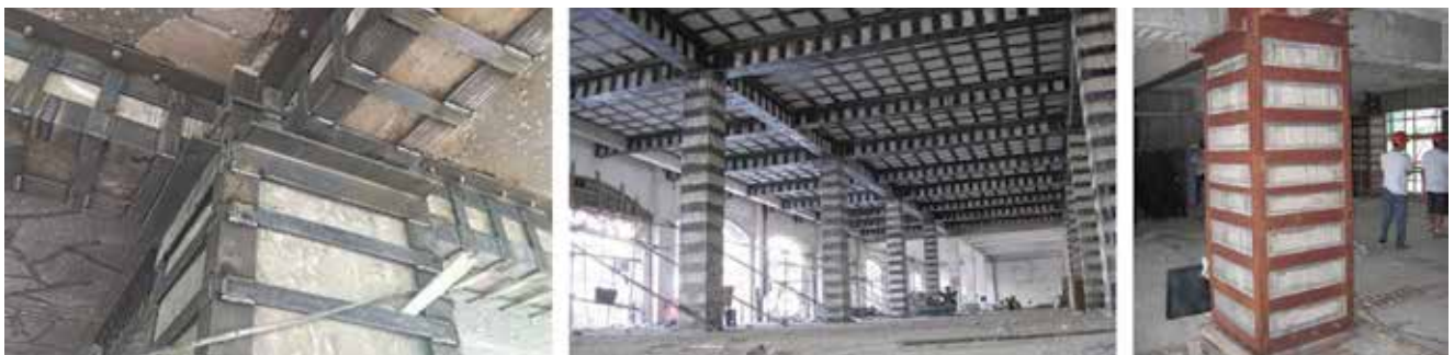
Figure 10. Retrofitting reinforced concrete members using steel plates
