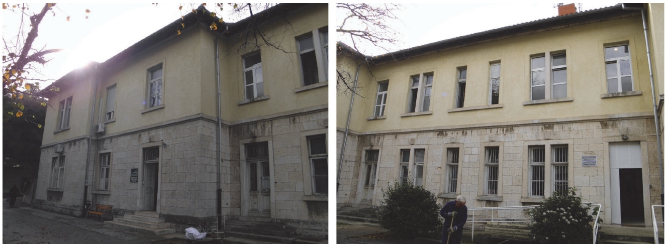
Figure 1. Old infectious disease building scheduled for demolition at Zadar General Hospital
