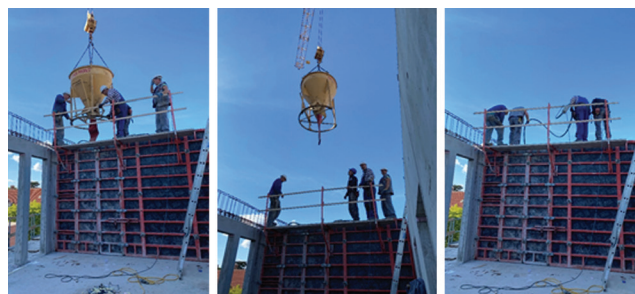
Figure 8. Casting recycled aggregate concrete for 3 rd floor walls of Zadar Day Hospital.
