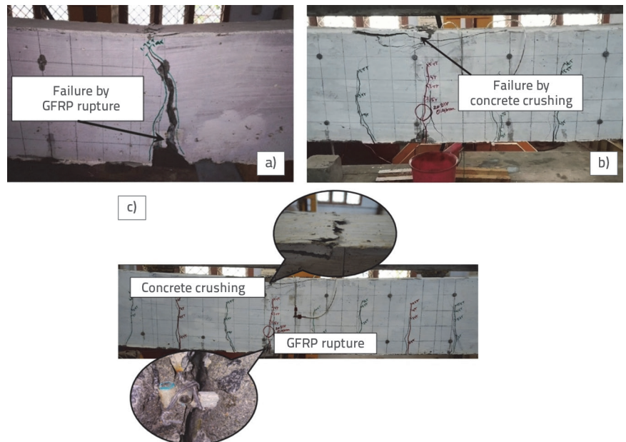
Figure 10. Typical failure mode of SCC beams: a) Under-reinforcement; b) Over-reinforcement; c) Balanced-reinforcement
