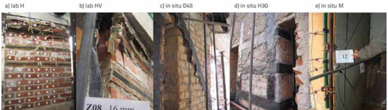
Figure 19. Failure modes of FRP reinforced masonry observed during testing
